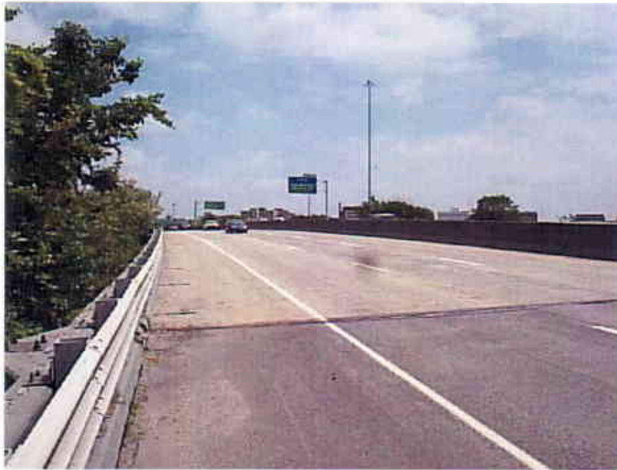
Photograph 13 View Looking East at the Top of the West Bound Lanes of the Interstate 90 Bridge over Ramps E-10 and E-8 (CUY-90-1640)
