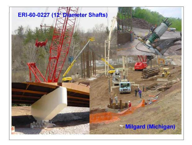
Figure 9.6: Example of a drilled shaft tied back for resistance of lateral soil forces
