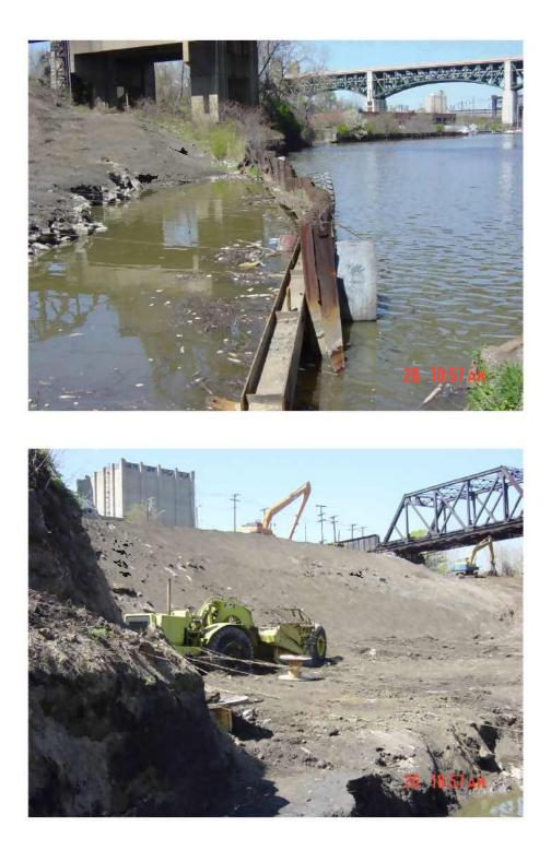
Figure 3.1. Pictures showing the failed sheet pile wall.
