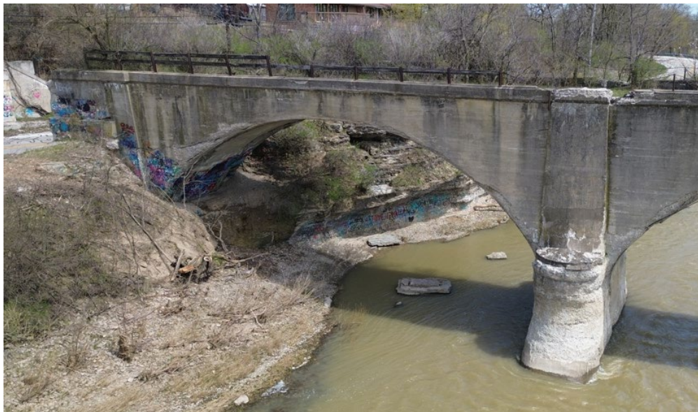
North end span (looking downstream) showing sound spandrel wall
