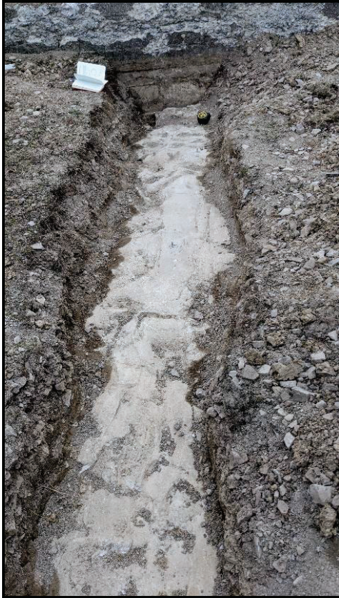
Photo 6 – Arch Extrados Exposed, Span 3.
