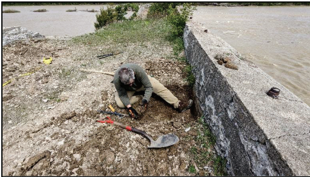
Photo 1 – Excavation of Span 3 Arch Intrados, May 3, 2026.
