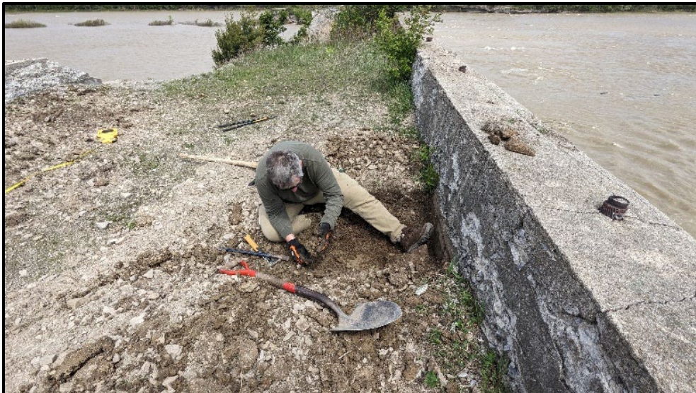
Photo 1 – Excavation of Span 3 Arch Intrados, May 3, 2026.
