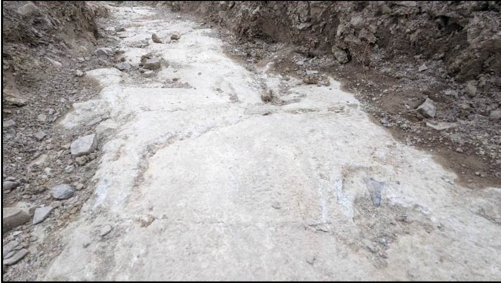
Photo 7 – Close-Up of Trowel-Finish and Good Condition of Arch Extrados Exposed, Span 3.
