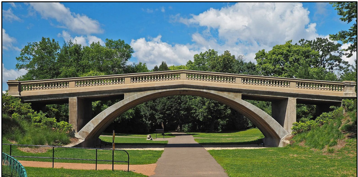
Photo 1 – Restored Interurban Bridge, Como Park, June 2024.
