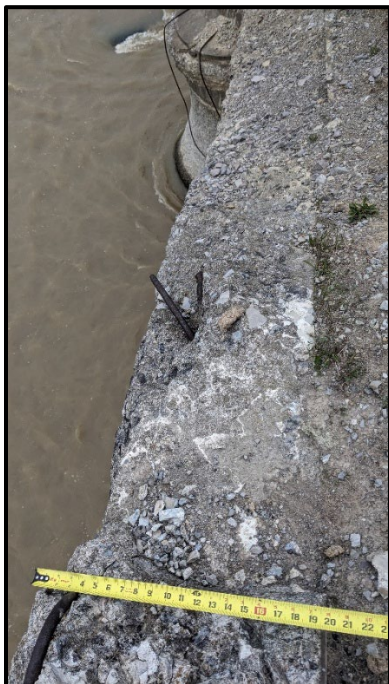
Photo 2 – Sparse Spandrel Wall Reinforcement, Span 2 East Spandrel Wall/
