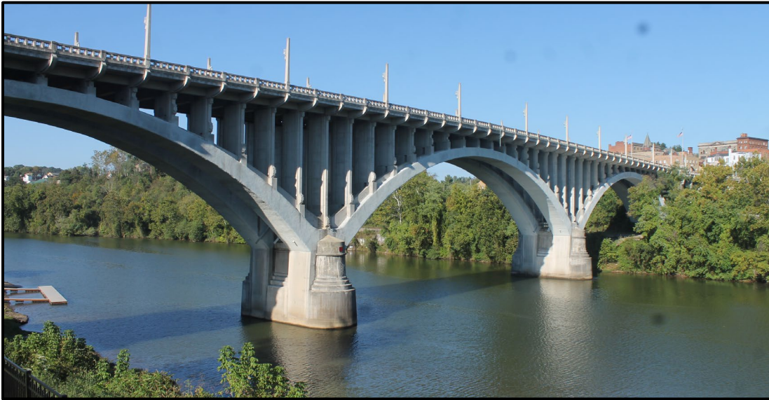
Photo 9 – Restored Jefferson Street Bridge, October 2016.
