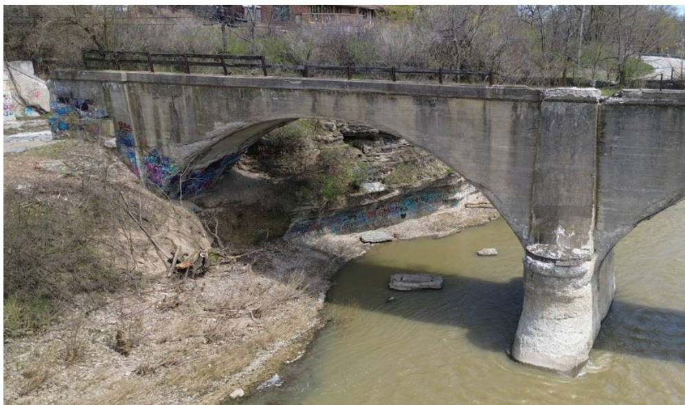
North end span (looking downstream) showing sound spandrel wall
