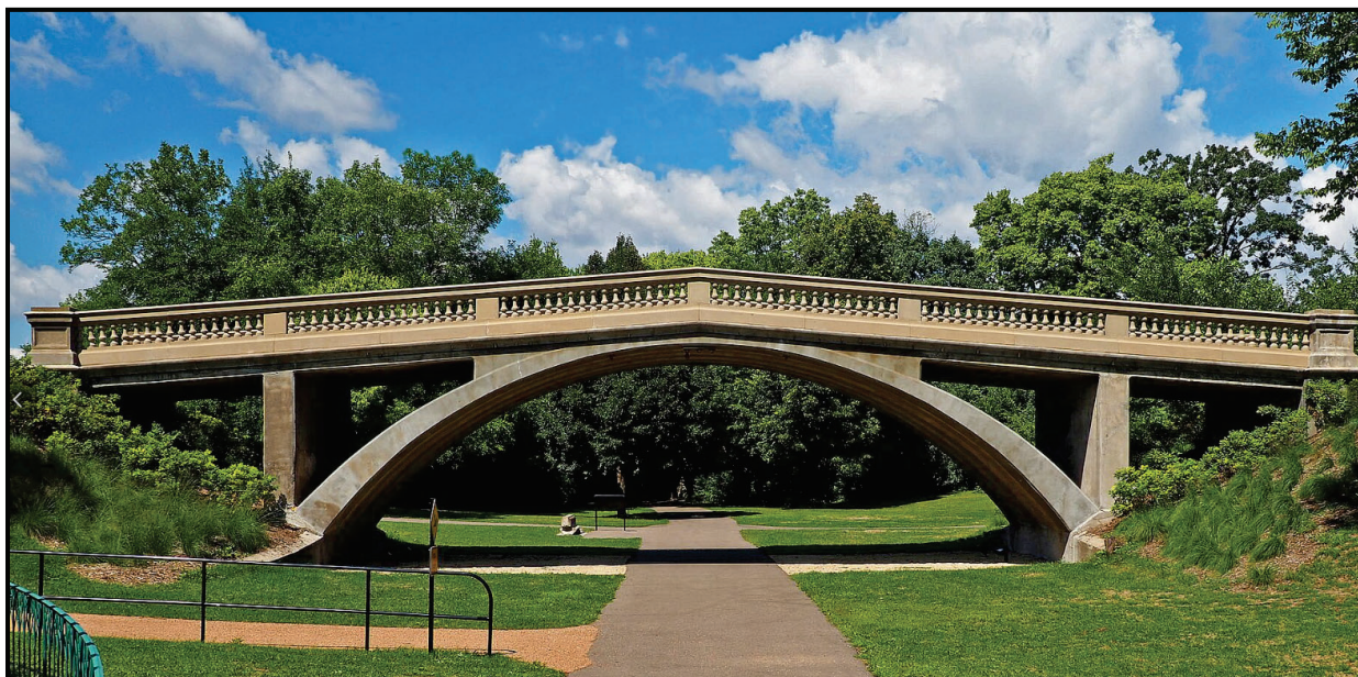
Photo 1 – Restored Interurban Bridge, Como Park, June 2024.
