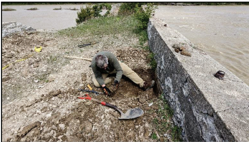
Photo 1 – Excavation of Span 3 Arch Intrados, May 3, 2026.
