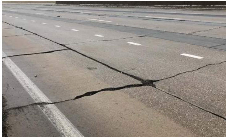
Photograph 5: Ramp P Concrete Pavement
