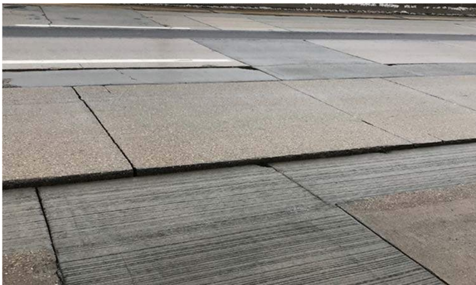
Photograph 2: IR-77 Pavement (Concrete)
