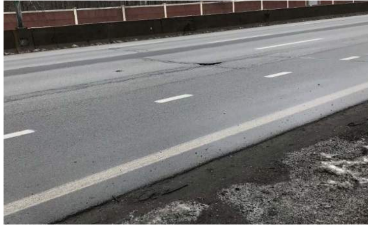
Photograph 3: IR-77 Pavement (Concrete)
