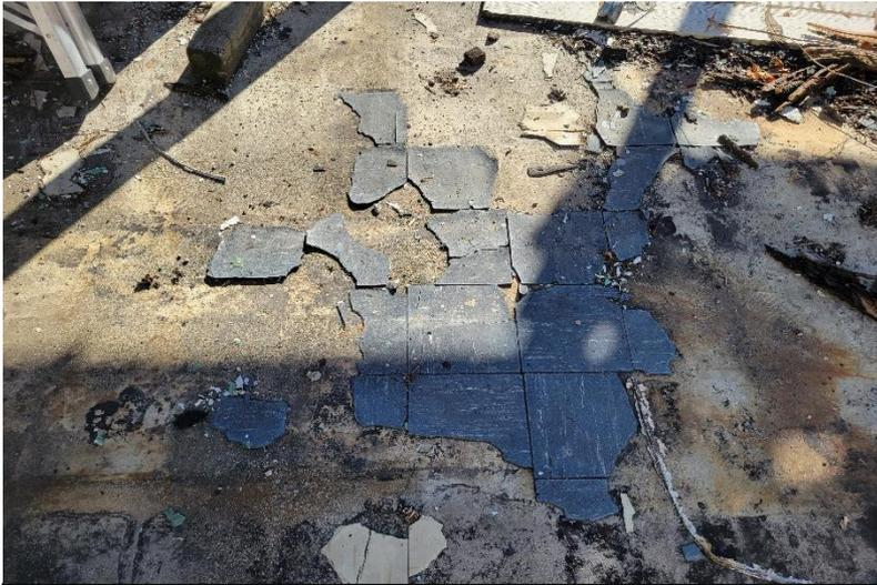
Photo 1 – View of asbestos-containing black floor tile in the concrete structure.
