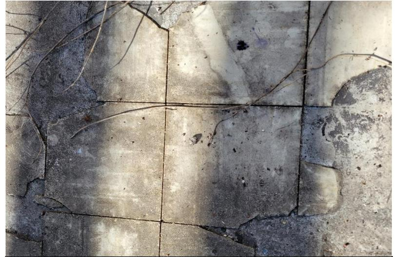
Photo 2 – View of asbestos-containing tan floor tile in concrete structure.
