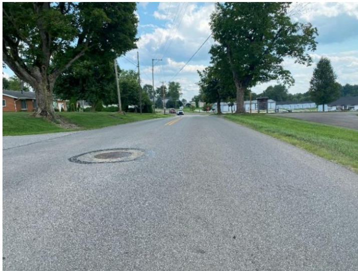
Picture 6: Looking SB on Upper Fredericktown Road approximately 325' north of North Sandusky Street (SR 13)
