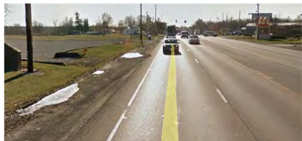
PHOTO 1: AGGEGATE SHOULDER WIDTH (EAST SIDE OF US ROUTE 23)
