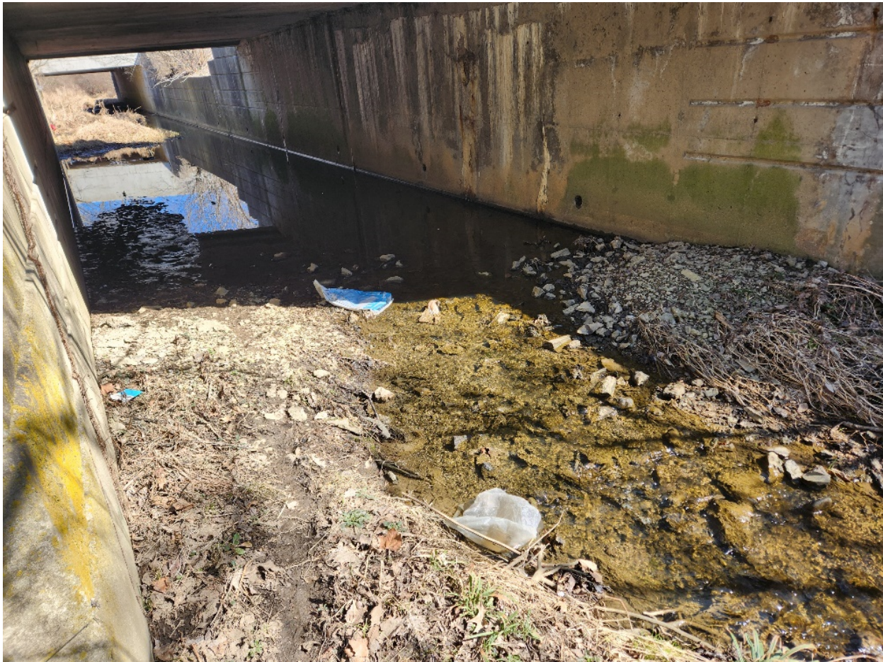
Figure 2: Bridge Opening Looking Upstream
