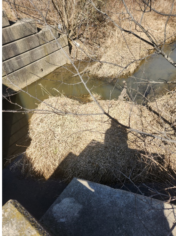
Figure 3: Upstream Bridge Opening
