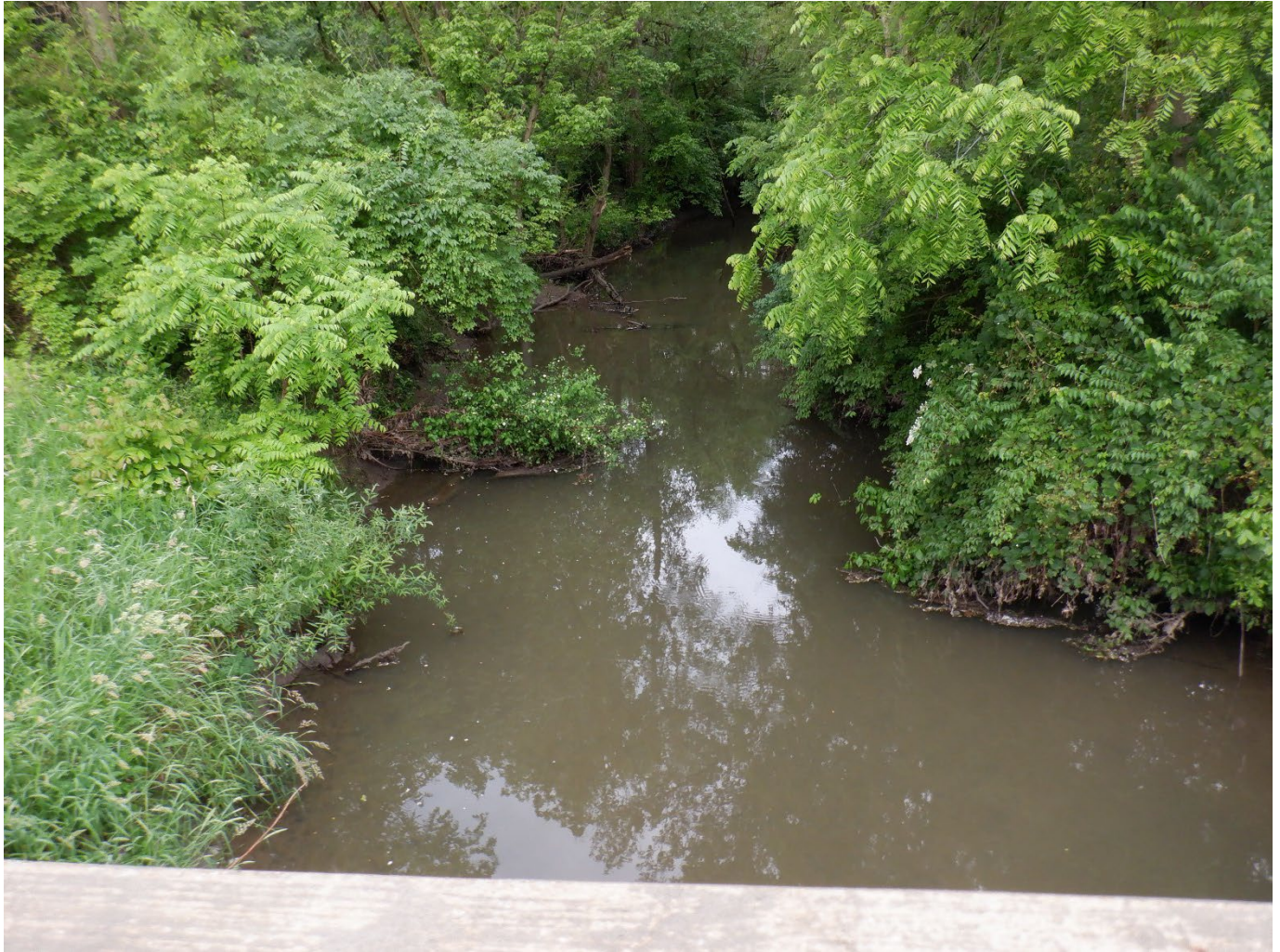
Georges Creek – Downstream Channel (Looking Downstream from Eastbound Existing Structure)
