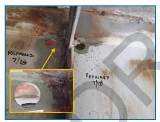
Photo 13 – Typical crack arrest hole in the web of Girder C near top flange (looking west in Span 23A at midspan).
