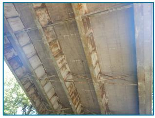
Photo 2 – Typical transverse cracks throughout the deck underside in the interior bays in Span 24A (looking northwest).
