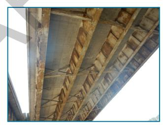
Photo 16 – Typical steel protective coating condition of all steel members in Span 21A (looking southwest).
