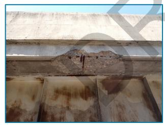
Photo 4 – 36" long by 24" wide by 4" deep spall with exposed reinforcement in the east overhang in Span 22A (looking west).
