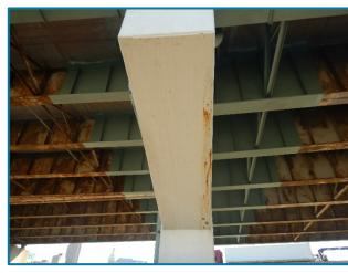
Photo 26 – Area of delamination, cracking, and rust staining on the underside of the Pier 19A cap (looking east at the west end of the cap).
