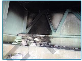
Photo 27 – Fire damage with discoloration and cracking on the Abutment A backwall between Girders C and D (looking northwest).
