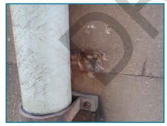
Photo 21 – 6" diameter spall near the drainage support bracket on the south face of Column 1 at Pier 23A (looking north about 15' above the ground).
