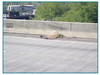
Photo 9 – Clogged scupper in the west shoulder on the top of deck at Pier 23A (looking southwest).
