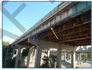
Photo 31 – Conduit along the exterior bottom flange of Girder A (looking northeast).
