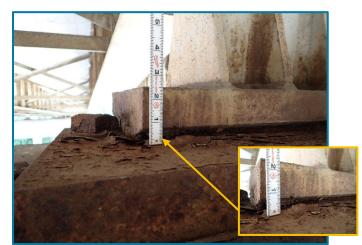
Photo 12 – 1/4" thick pack rust between the masonry plate and rocker bearing of Girder E at Pier 20A (looking southwest).
