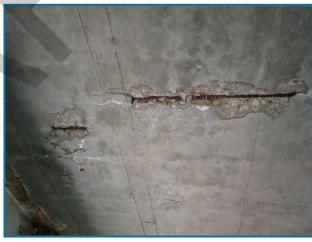
Photo 1 – Isolated delamination/spall with exposed reinforcement and adjacent typical hairline transverse cracks in the deck underside (looking up and south between Girders B and C in Span 23A).
