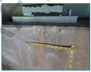
Photo 24 – Shallow edge spall on the Abutment A bearing seat at Girder D (looking north).
