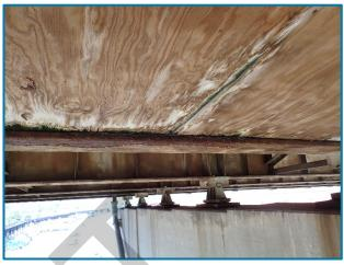
Photo 11 – Laminate corrosion with up to 1/8" section loss in the bottom flange of Girder E in Span 20A near Pier 20A (looking east).
