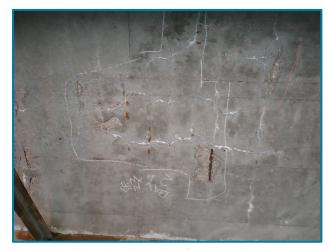
Photo 5 – 8' long by 8' wide by 1" deep spall with exposed reinforcement and surrounding delaminations in the deck underside between Girders B and C in Span 23A (looking south).
