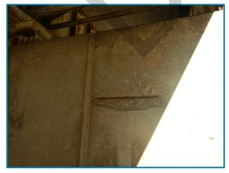
Photo 25 – 2' wide by 1' high by 2" deep spall with exposed reinforcement on the south face of the Pier 21A cap between Girders D and E (looking north).
