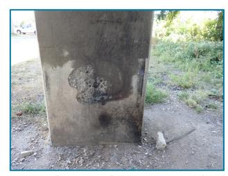
Photo 22 – 20" diameter by 1" deep spall on the north face of Column 2 at Pier 23A (looking south near the base).
