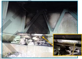
Photo 18 - Fire damage to the end crossframe between Girders C and D at Abutment A (looking northwest).
