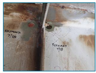
Photo 19 – Typical crack arrest hole repairs in east face web of Girder C at the midspan crossframe connection (looking west in Span 23A).
