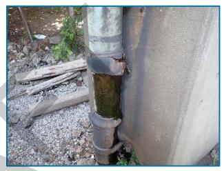
Photo 10 - Bulging and cracked drainage coupling gasket at the base of Column 1 on the south face of Pier 23A (looking northwest).
