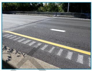
Photo 28 – New asphallt wearing surface overlay on the north approach slab (looking southwest).
