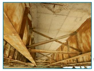
Photo 17 – Typical crossframe with minor surface corrosion and paint failure (looking south in Span 21A between Girders D and E).
