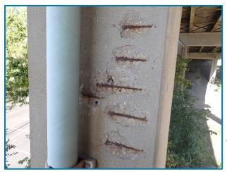
Photo 20 – Spalls with exposed reinforcement on the south face of Column 1 at Pier 22A (looking north).
