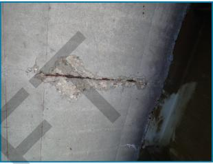
Photo 3 – 24" wide by 12" long by 1" deep spall with exposed reinforcement in the deck underside between Girders D and E in Span 24A (looking south).
