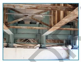
Photo 15 – Typical steel protective coating condition of the girder ends at Pier 19A (looking southeast).
