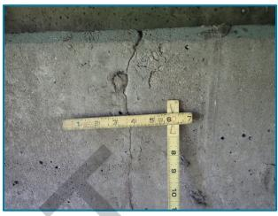
Photo 23 – Isolated vertical hairline crack in the abutment seat below Girder B in Span 25A (looking north at the south face of Abutment A).
