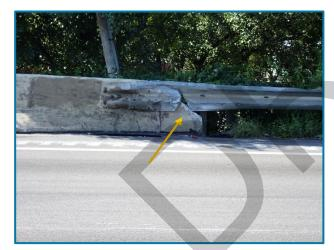
Photo 29 – Impact damage to the approach guardrail at the transition to the concrete railing on the west side of the north approach (looking west). Note the spall at the end of the concrete railing.
