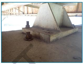
Photo 14 – One broken anchor bolt at the northeast corner of the Girder C bearing at Pier 22A (looking southwest).
