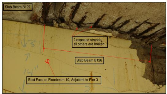
Photo: Western End of Slab Beam B126 at Pier 3
