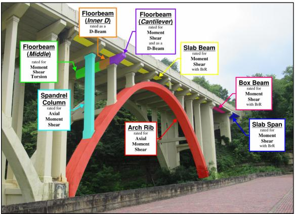
Figure F. Representative Graphic with Location and Type of Load Ratings
